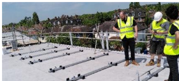
Work in progress on a school installation
